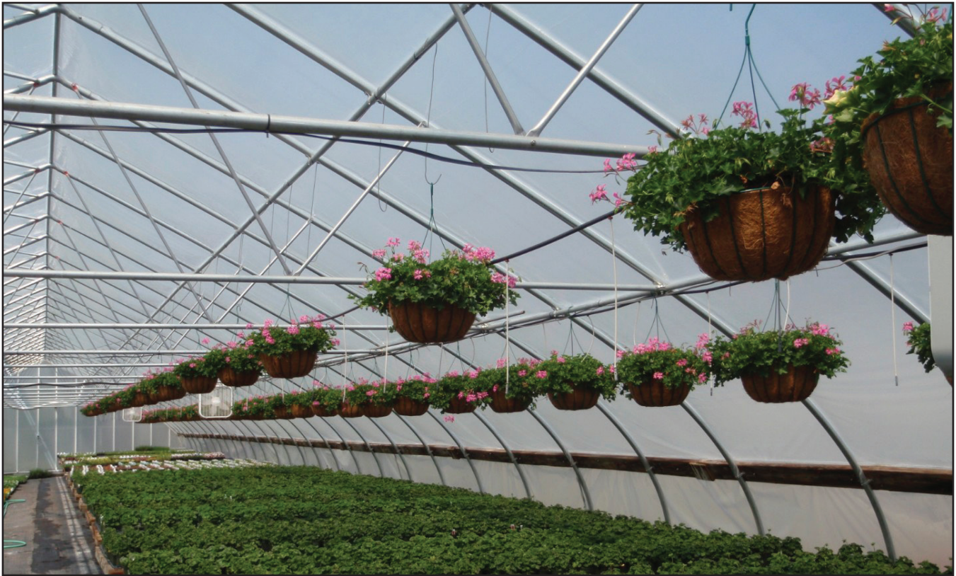
Figure 4. Proper spacing of baskets above crops on benches
